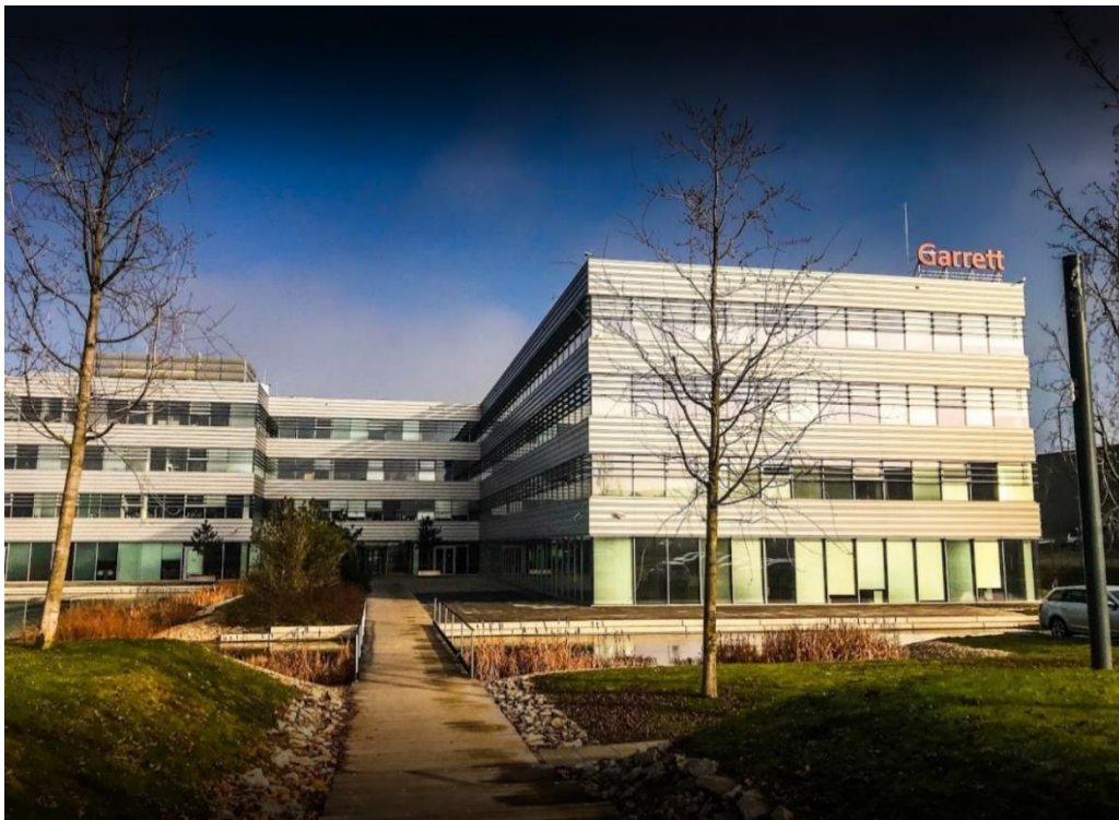
Obr. 4: Budova Garrett v Brne [4]
